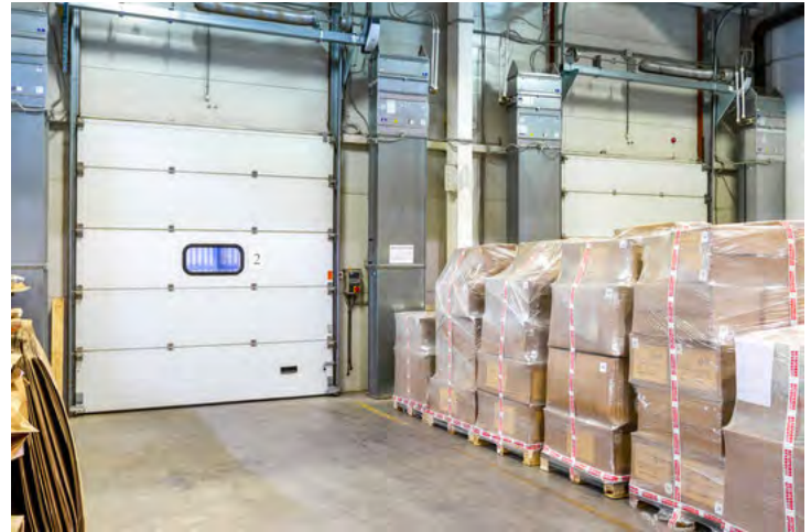
Indoor staging area at loading dock with sealed concrete floors and minimal finishes
