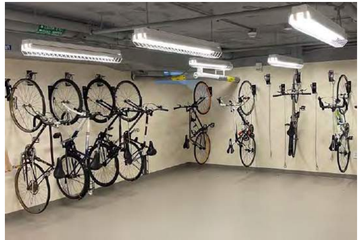
Winthrop House, Harvard - Wall based bicycle hangers with integrated cable locks
