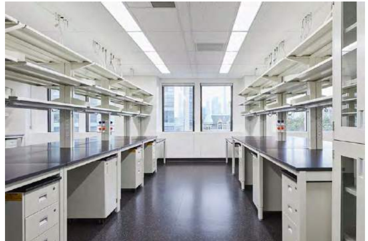
Medical Sciences Building, UoT - Standardized isolated workstations, ceiling based service distribution, and acoustic ceiling treatment
