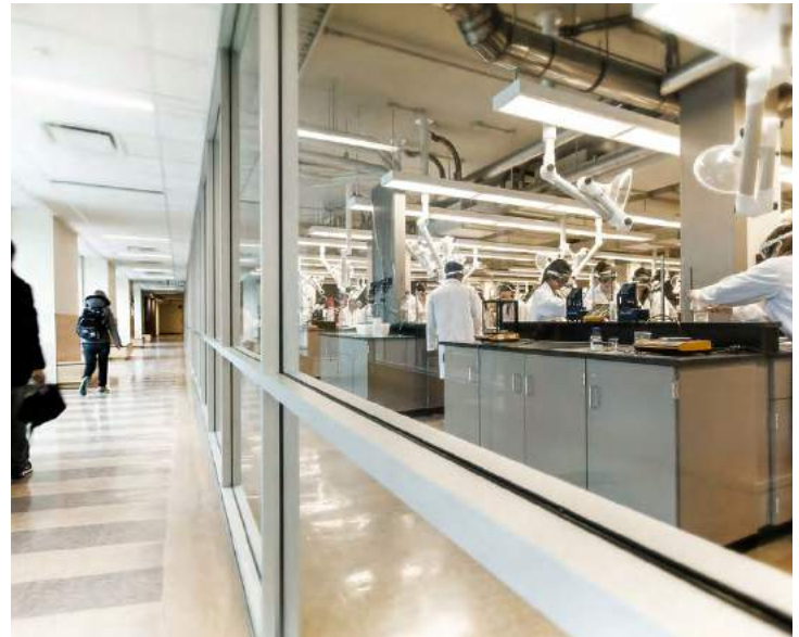
Chernoff Hall Lab, Queens - Lab with extension arm fume extractors and high transparency to the corridor providing visual activation
