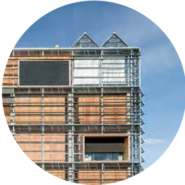
ICTA-ICP Building, Autonomous University of Barcelona, H Arquitectes & DATAAE
